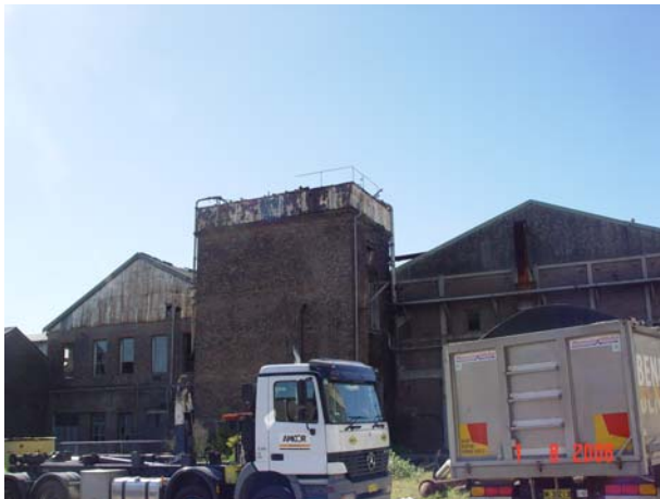
Derelict buildings that have already been removed
