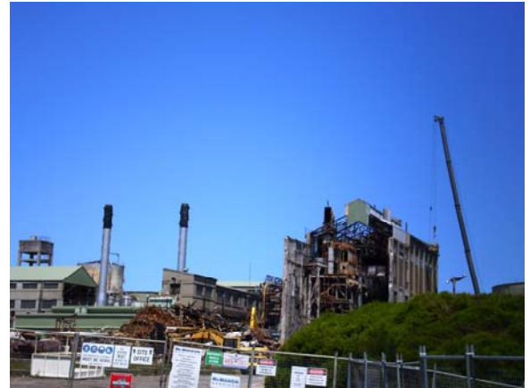
Buildings currently being demolished
