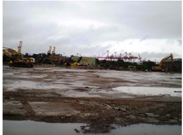
A photo of the now bare concrete slab
